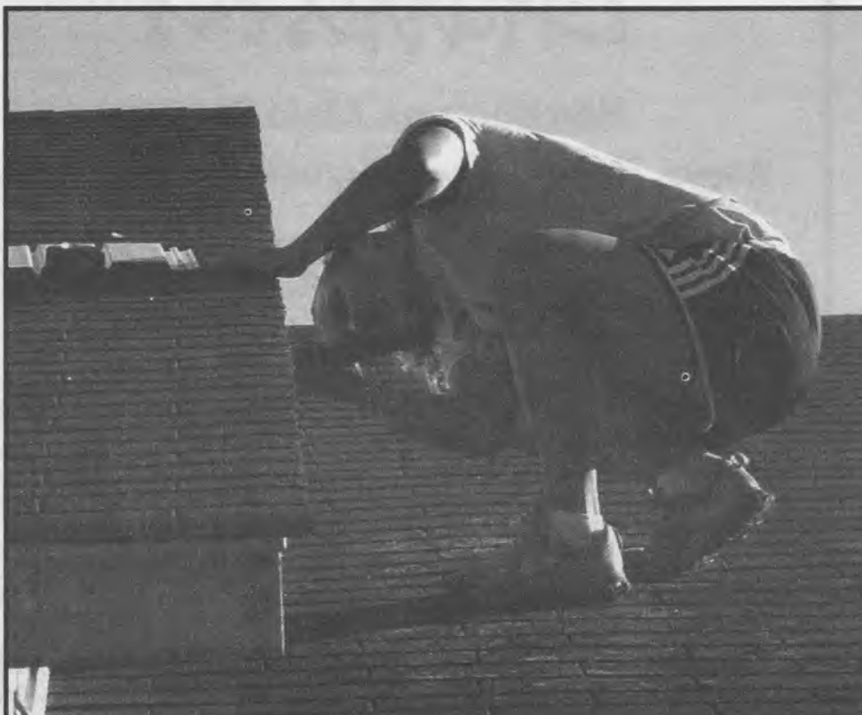
APO member Mary Beth Long, sophomore, applies siding to a house on a Habitat for Humanity trip to Tupelo, Miss. during fall break. Photo by Dan Costello
